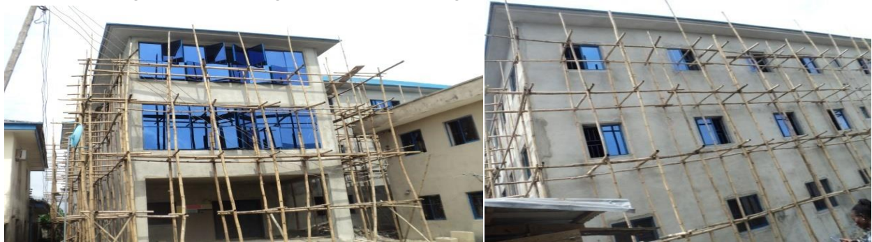
Picture 44: The Medical Records Block almost completed at FMC Yenagoa
