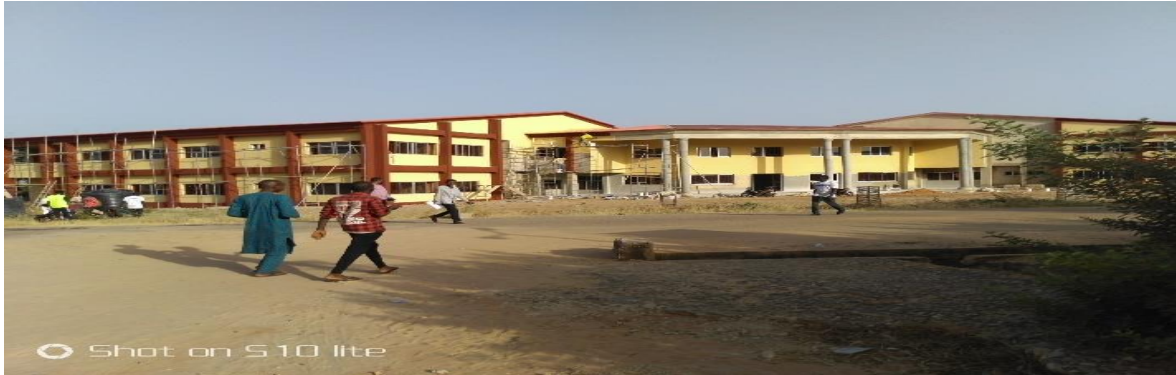
Picture 36: Ongoing construction of Agric. Complex
