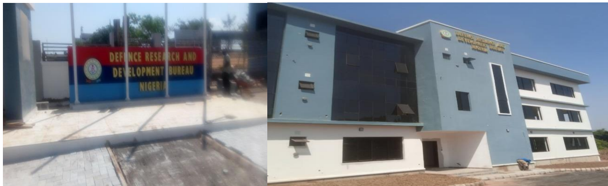
Picture 9: The Completion of the construction for 2-storey complex DRDB headquarters Annex building and Gatehouse.
