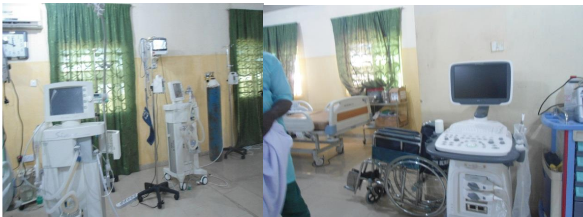
Picture 50: Some of the Medical Equipment Procured and Installed at the ICU, FMC Zamfara
