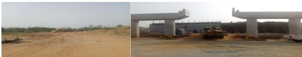
Picture 81: On-going bridge works at Inner Southern Expressway (ISEX) Project.
