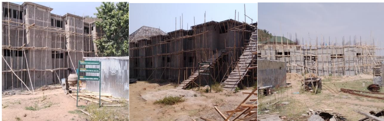
Picture 66: Ongoing Construction of Medium, Maximum and Dormitory Cells at Karshi-Abuja
