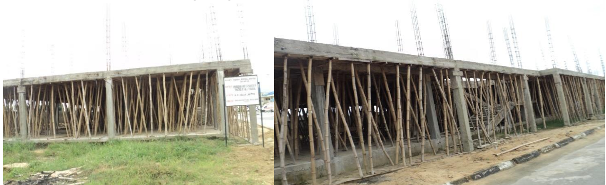
Picture 45: Ongoing construction of 6-theatre suites building at FMC Yenagoa
