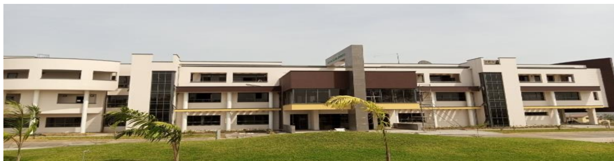
Picture 67: Construction of Technology Building at Nigerian Immigration Service Headquarters, Abuja
