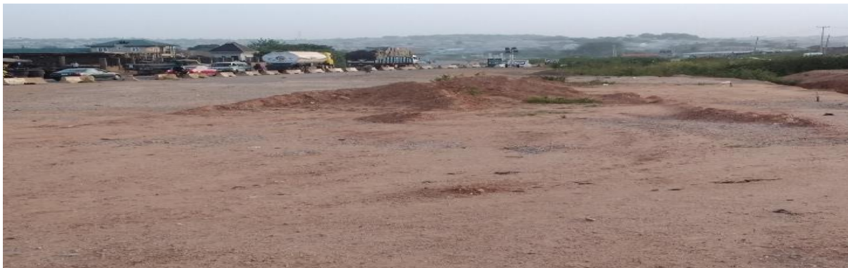
Picture 3: Ongoing earthworks at Ibadan-Ilorin Road, Section II: Oyo-Ogbomosho
