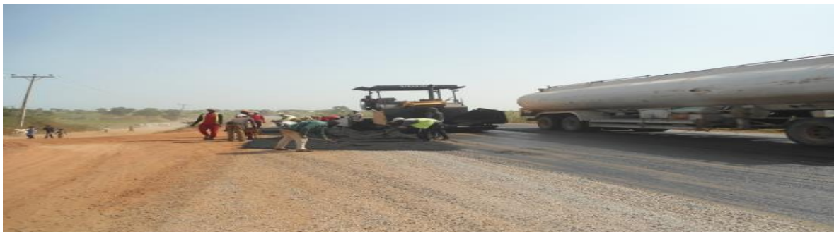
Picture 6: Ongoing asphalt and scarification works at Yauri town
