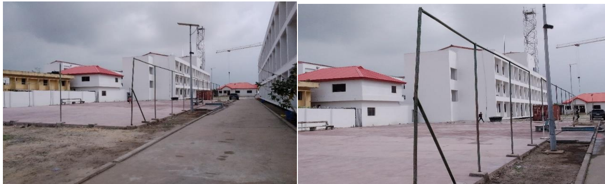
Picture 60: Completed Students' Hostel at FCFMT, Lagos
