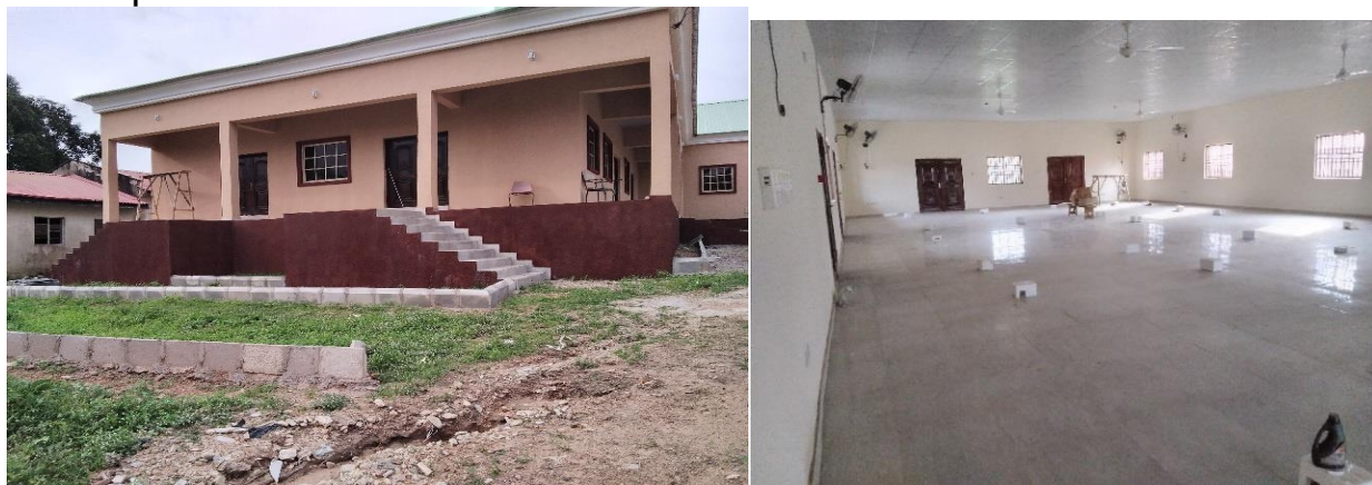
Picture 76: On-going Construction of Computer Laboratory
