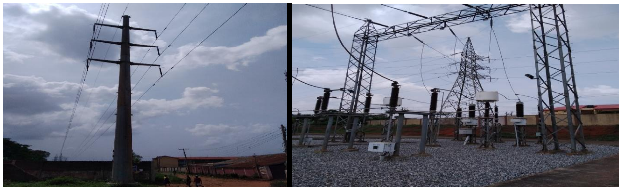
Picture 30: Completed tower lines at Ikorodu-Odogunyan-Sagamu
