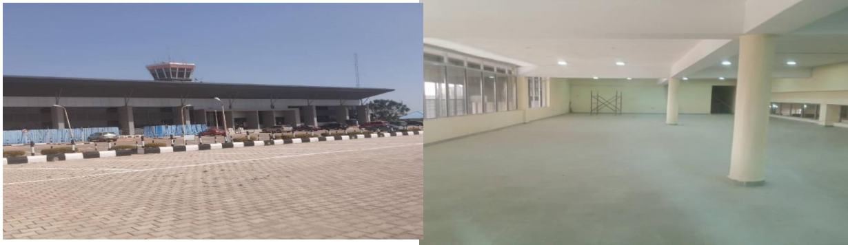
Picture 28: On-going Upgrade and Rehabilitation of Jos Airport Terminal Building.
