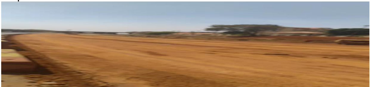
Picture 80: Ongoing Earthworks at the Outer South Expressway (OSEX) Phase 1
