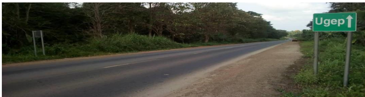
Picture 7: Ongoing Rehabilitation of Alesi-Ugep Section in Cross River State
