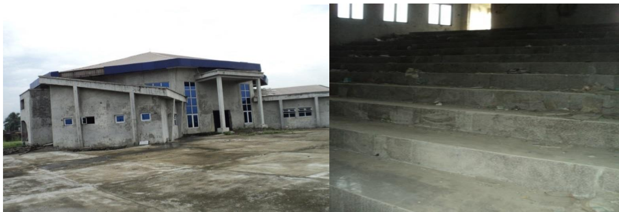
Picture 62: Construction of 300-Seater Lecture Theatre & External Works at PTI, Effurun
