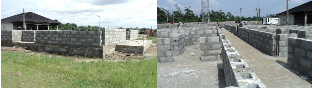
Picture 33: Construction/Provision of Hostel in progress at Nigeria Maritime University, Okerenkoko
