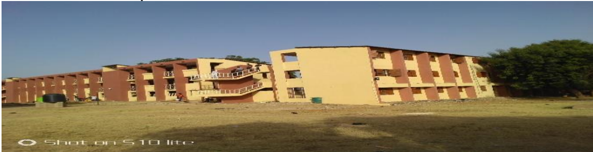
Picture 37: Completed Rehabilitation of Male Hostels
