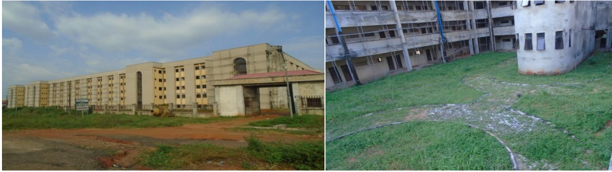
Picture 8: On-going Construction of Federal Secretariat Complex Awka, Anambra State
