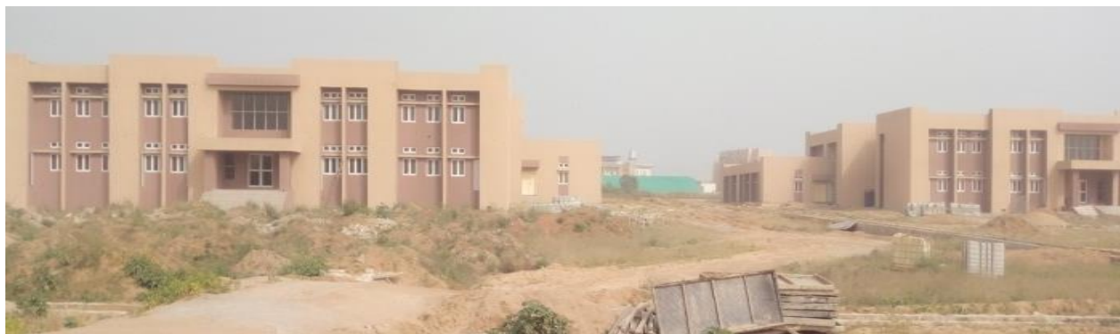
Picture 40: Completed 4-block buildings of Faculty of Veterinary Medicine at Bayero University, Kano
