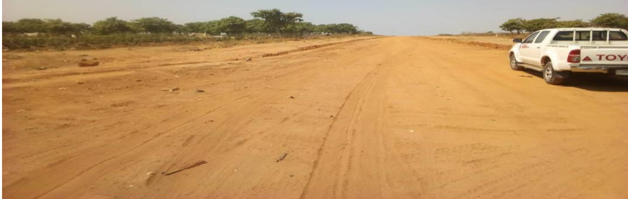
Picture 82: Ongoing Earthworks at the Inner Northern Expressway (INEX) Project
