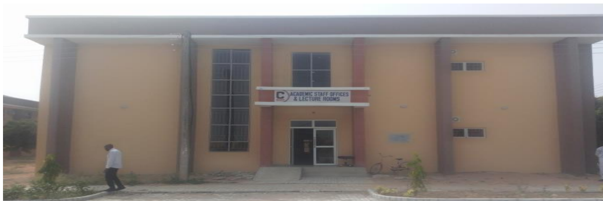
Picture 39: One of the 2nos. completed offices/lecture halls at College of Health Sciences, Bayero University, Kano.
