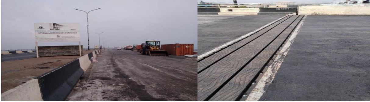
Picture 4: On-going Rehabilitation/Maintenance of Third Mainland Bridge in Lagos State
