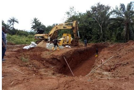
**Picture 9:** Ongoing palliative and culvert works at the Dualization of Akure – Ado Ekiti road project.
