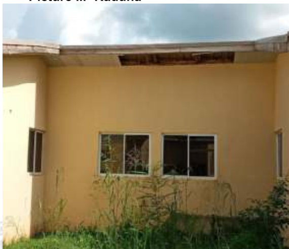
Picture III- Kaduna
