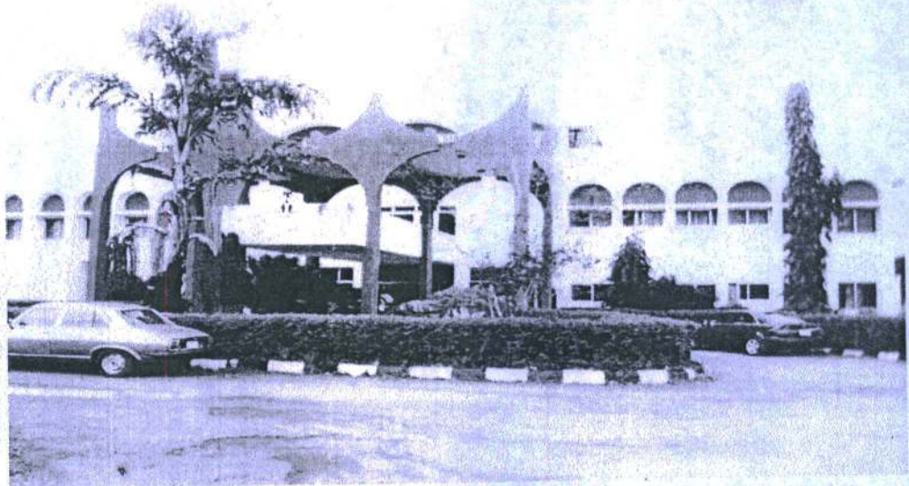
THE STATE HOUSE OF ASSEMBLY COMPLEX, REHABILITATED AND FURNISHED BY GOV. PETER OBI.
