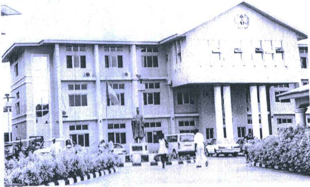
THE NEW ONITSHA NORTH LOCAL GOVERNMENT HEADQUARTERS
