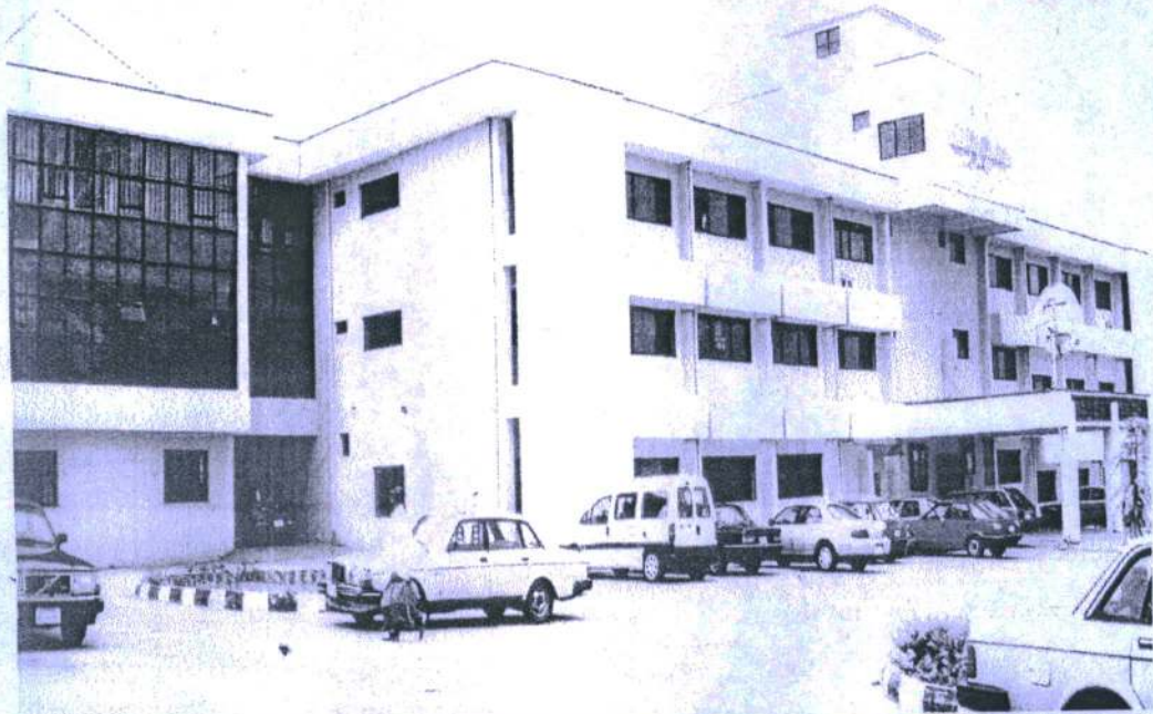
ANAMBRA STATE UNIVERSAL BASIC EDUCATION BOARD (ASUBEB) BUILDING COMPLETED BY GOVERNOR PETER OBI TO SUPPORT HIS ADMINISTRATION'S EDUCATION SECTOR PROGRAMME
