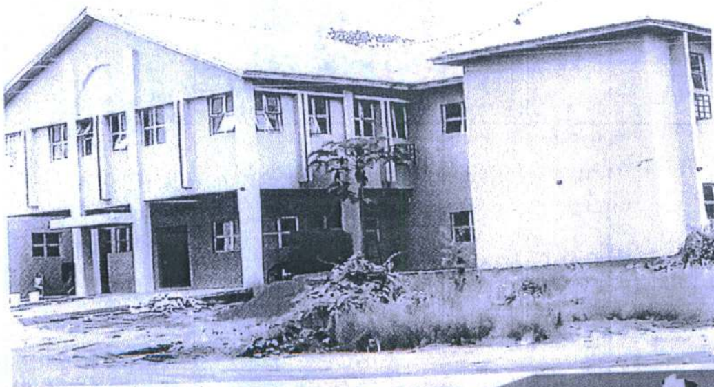
COMPLETED NEW AGUATA ZONAL OFFICE OF THE MINISTRY OF JUSTICE
