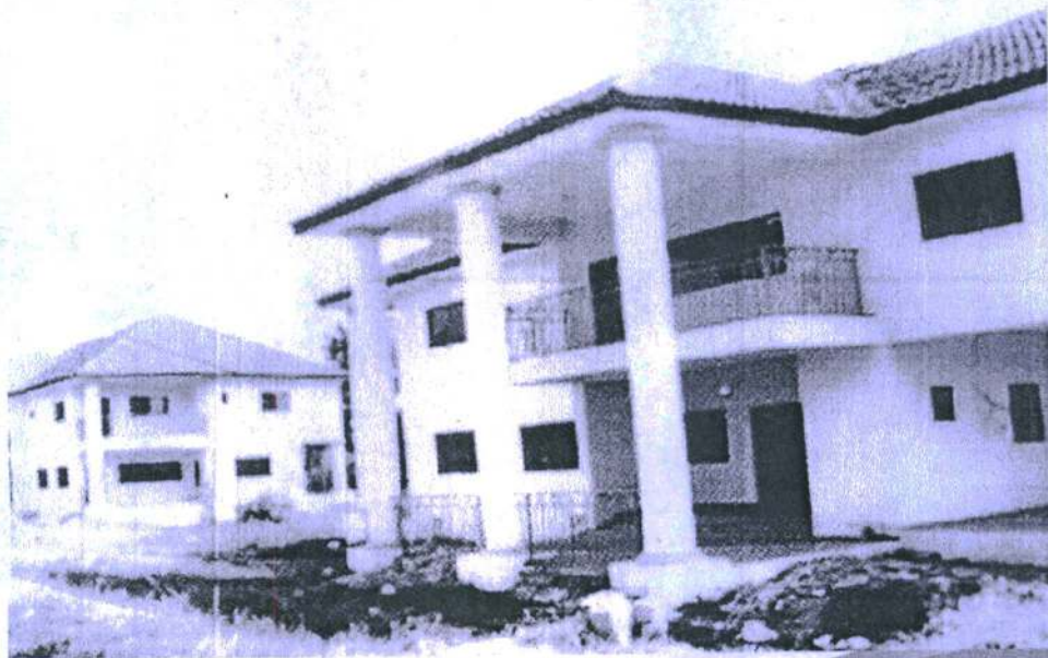
TWO OF THE MANY BUILDINGS AT JUDGES' QUARTERS, ONITSHA THE FIRST EVER IN THE STATE.
