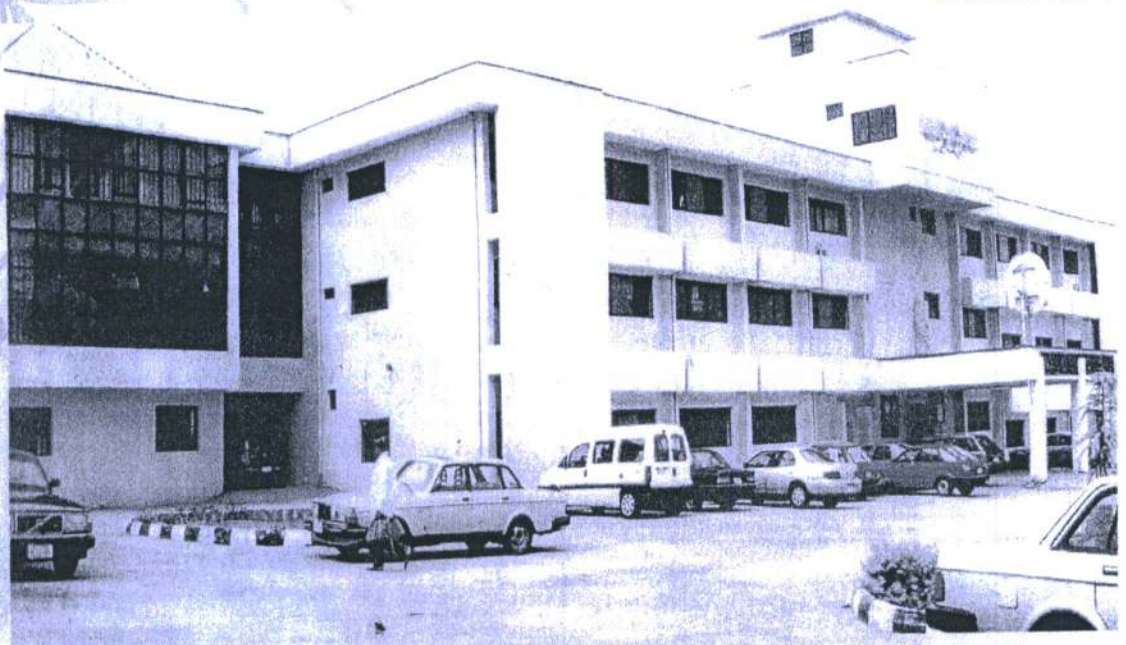
ANAMBRA STATE UNIVERSAL BASIC EDUCATION BOARD (ASUBEB) BUILDING COMPLETED BY GOVERNOR PETER OBI TO SUPPORT HIS ADMINISTRATION'S EDUCATION SECTOR PROGRAMME
