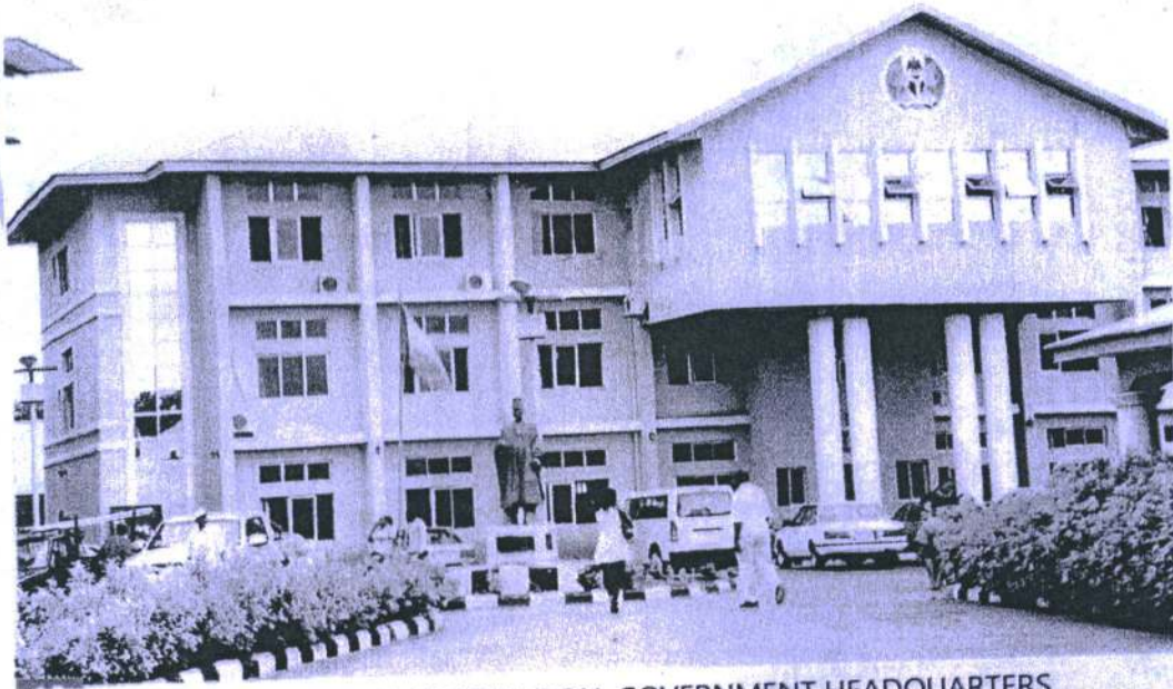
THE NEW ONITSHA NORTH LOCAL GOVERNMENT HEADQUARTERS
