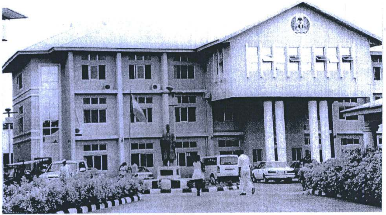
THE NEW ONITSHA NORTH LOCAL GOVERNMENT HEADQUARTERS
