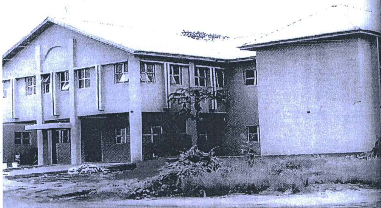
COMPLETE NEW AGUATA ZONAL OFFICE OF THE MINISTRY OF JUSTICE
