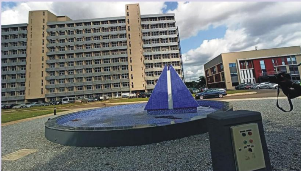
NEW SECRETARIAT BUILDING 2
