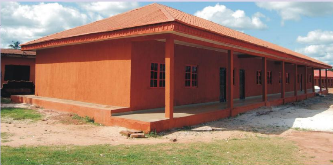
NEWLY CONSTRUCTED CENTRAL PRY SCH. UBIAJA
