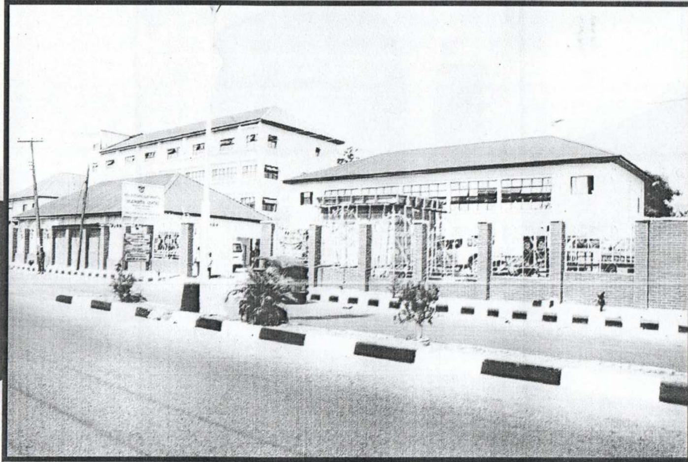
Construction of Diagnostic Centre Umuahia
