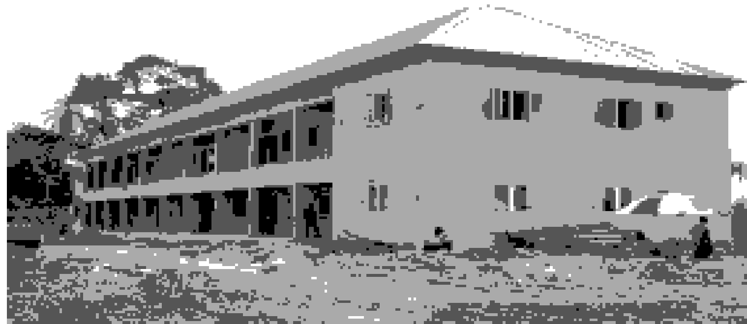
VOCATIONAL CENTRE SAMPOU ON-GOING
