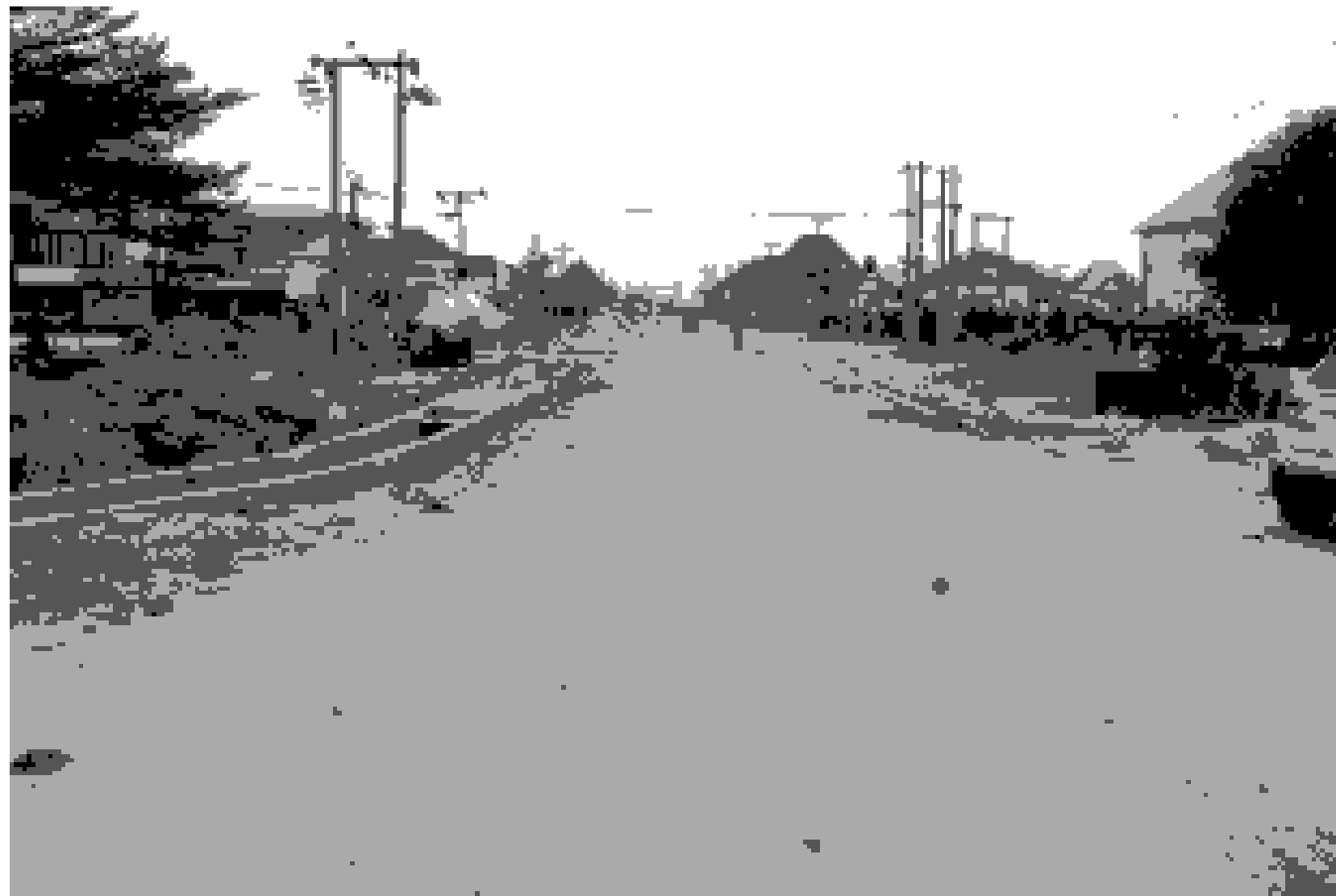
COMMISSIONERS ESTATE ROAD OPOLO ON-GOING
