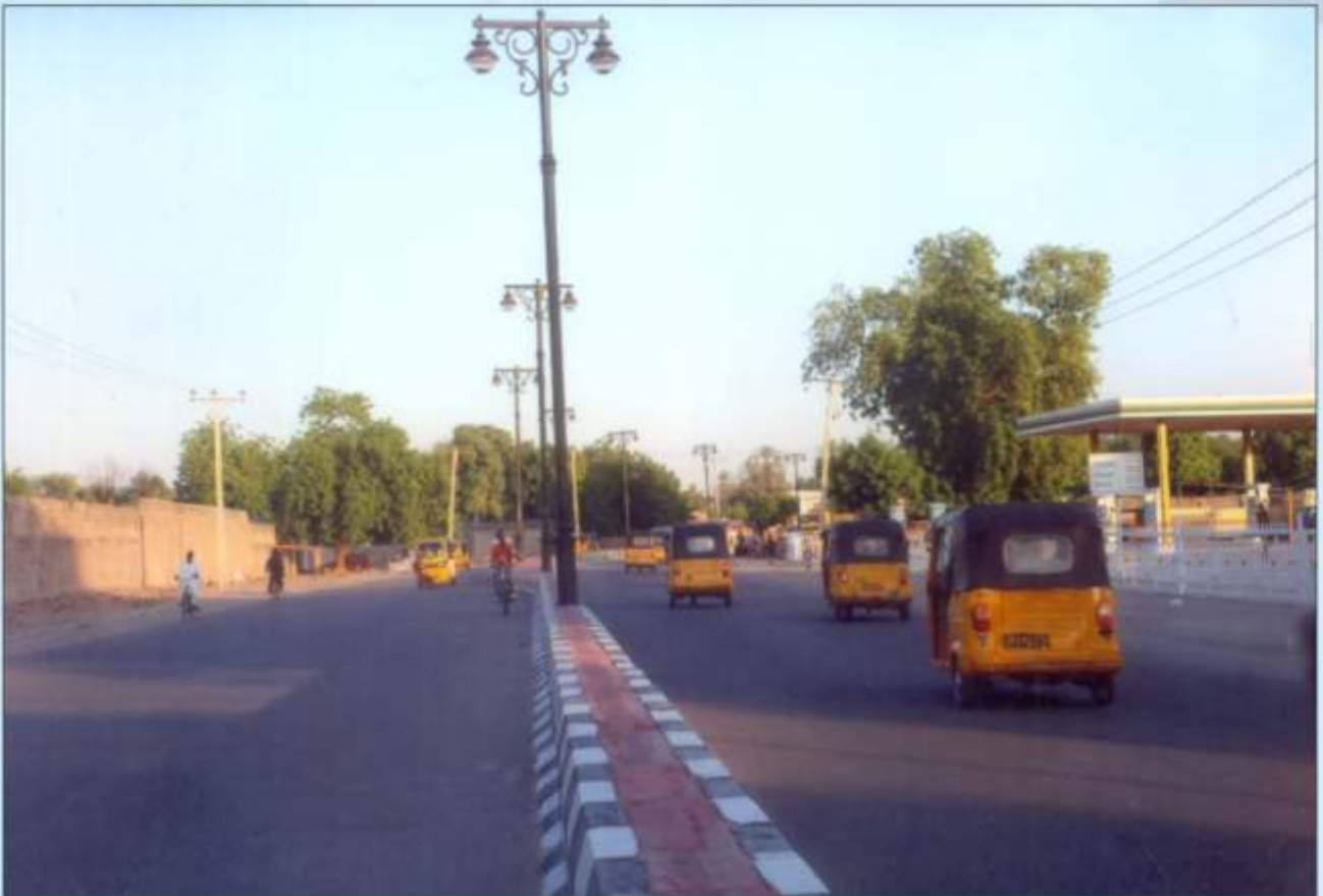
Reconstruction of Maiduguri Township Roads
