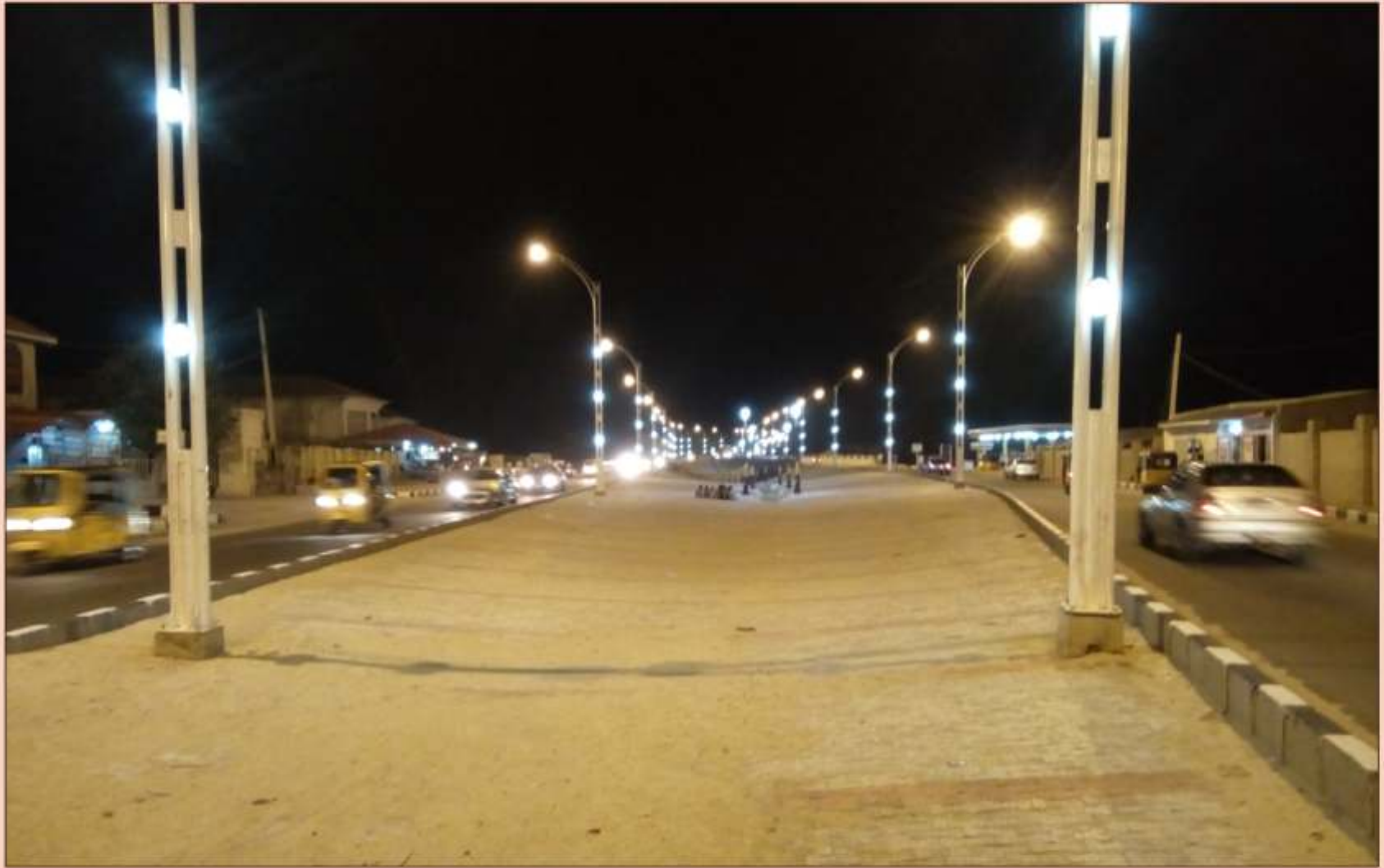
Night view of Dual Carriage Bridge, Lagos Street, Maiduguri
