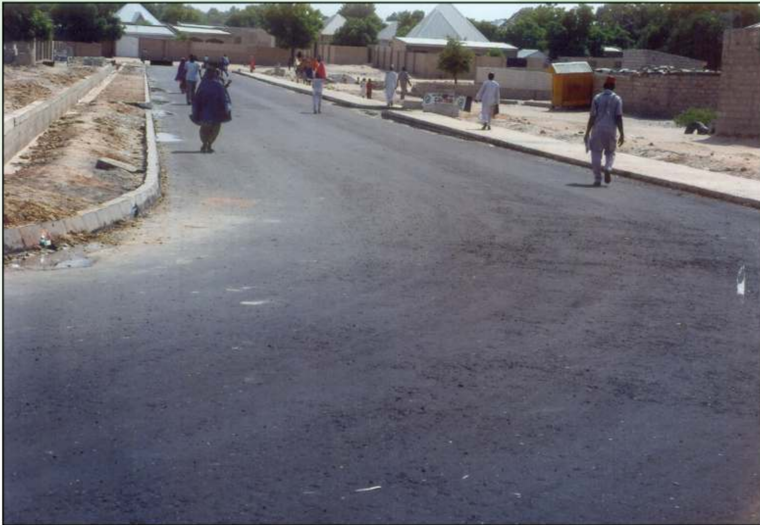
Fori - Galtimari Road Construction and Drainage, Maiduguri
