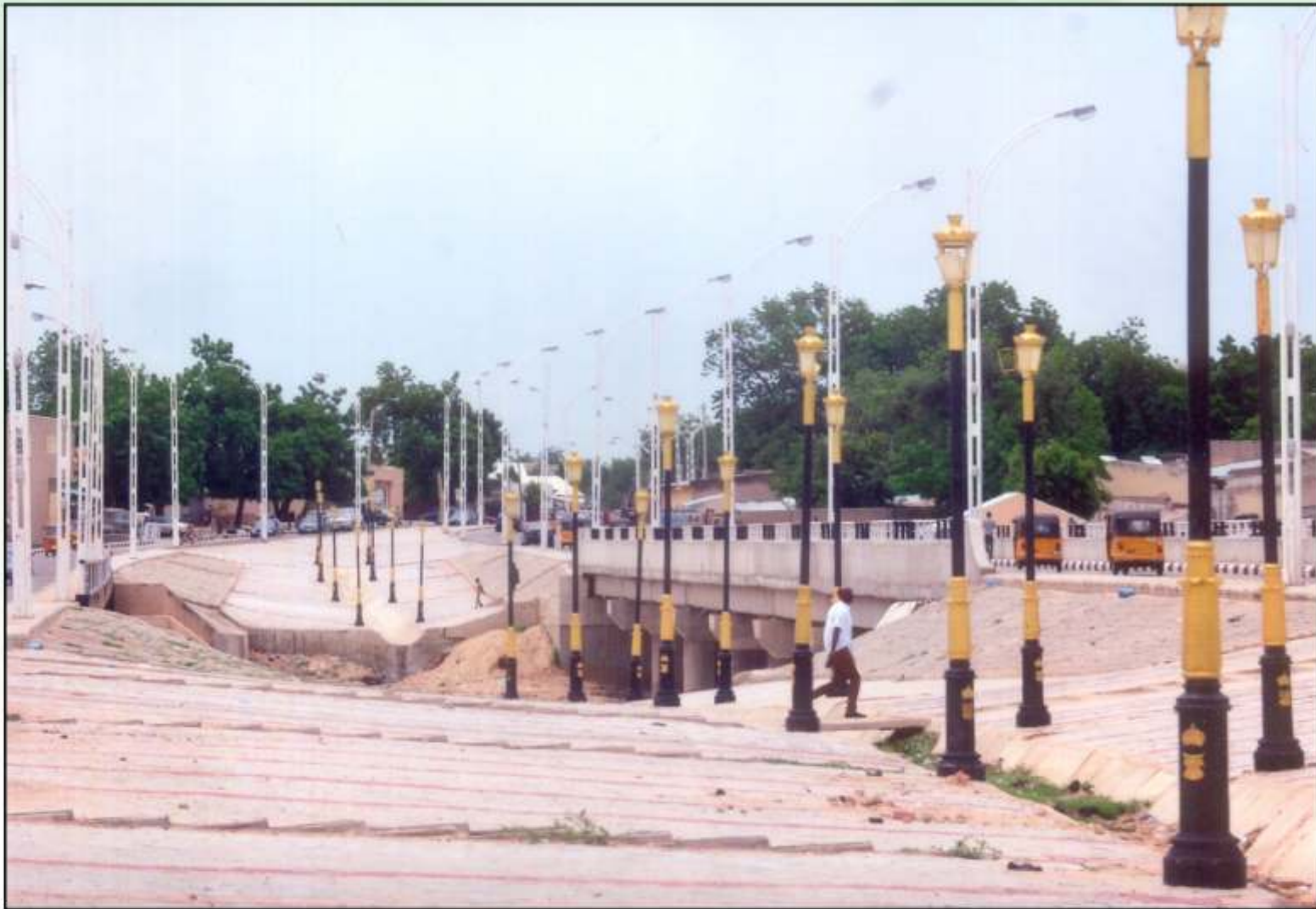
Dual - Carriage Bridge, Lagos Street, Maiduguri
