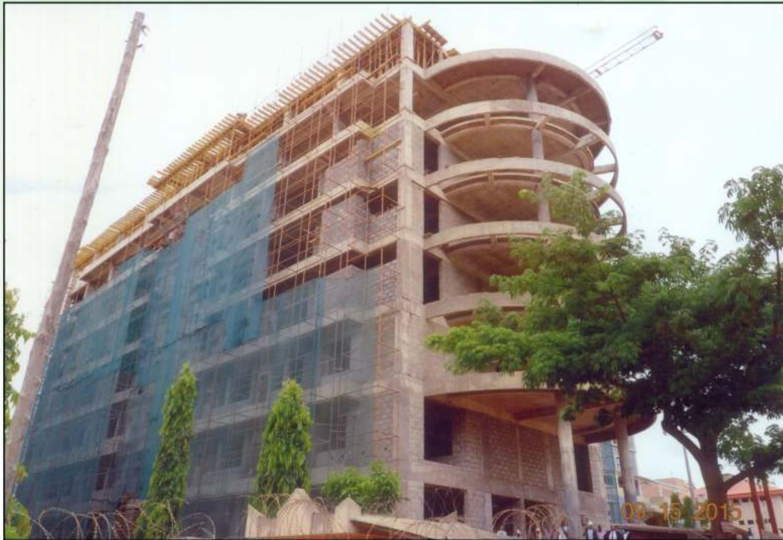
New Borno House Abuja Under Construction
