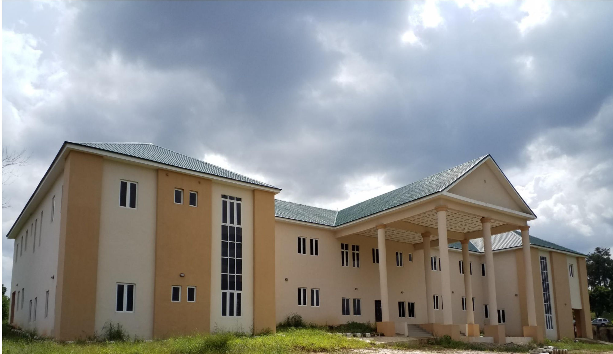
NEWLY CONSTRUCTED, COURT BUILDING
