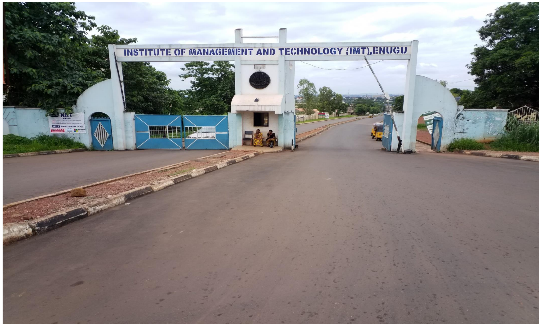
NEWLY REHABILITATED IMT ROAD
