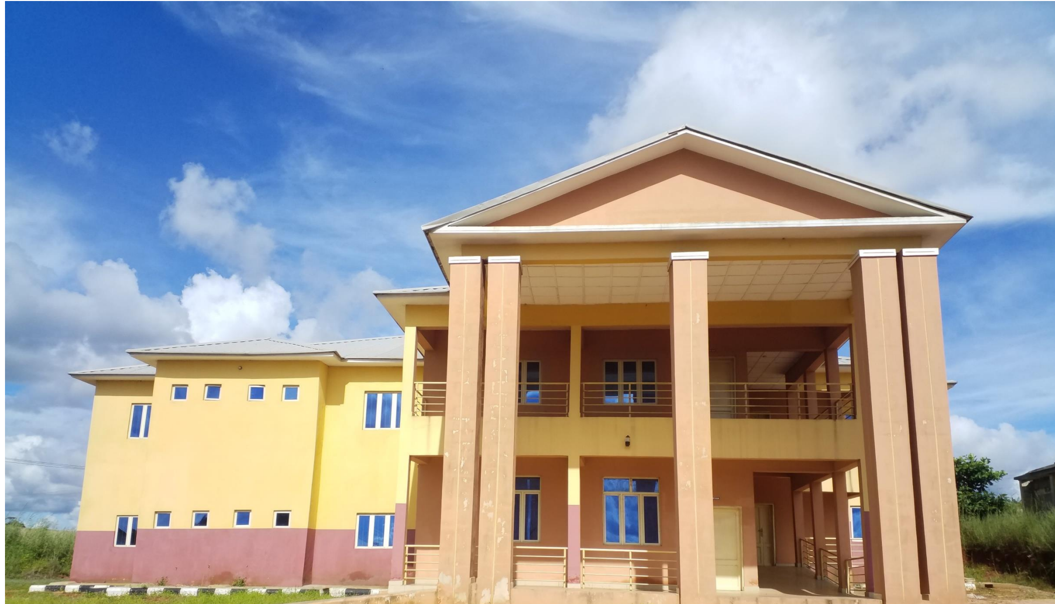
NEWLY CONSTRUCTED, STATE HOSPITAL MANAGEMENT BOARD, GENERAL HOSPITAL NSUKKA
