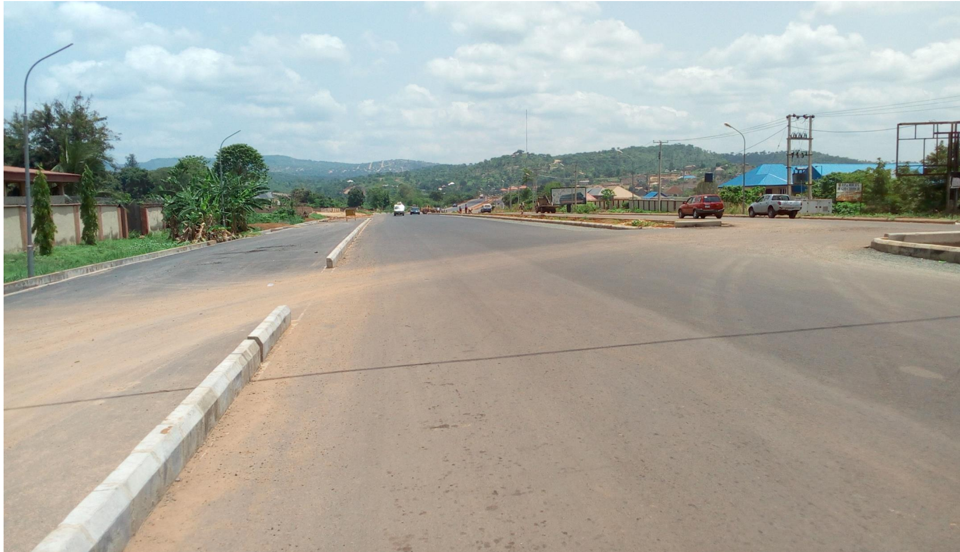
NEWLY CONSTRUCTED, AGUABOR INTERCHANGE SLIP ROAD-NEW MARKET
