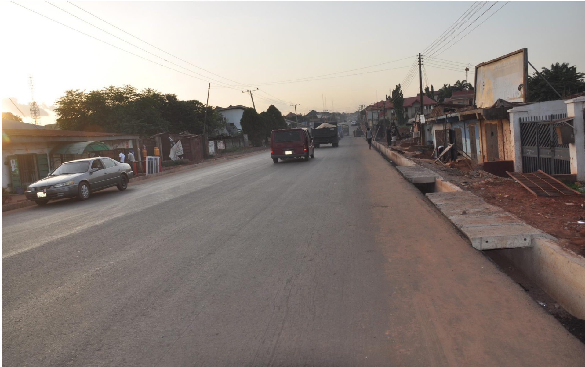
Nike Lake Road asphalted
