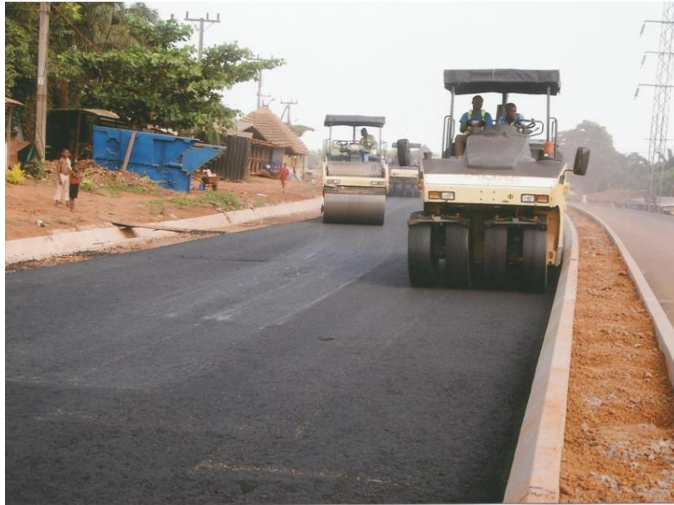
A PORTION OF NSUKKA URBAN ROADS BEING ASPHALTED
