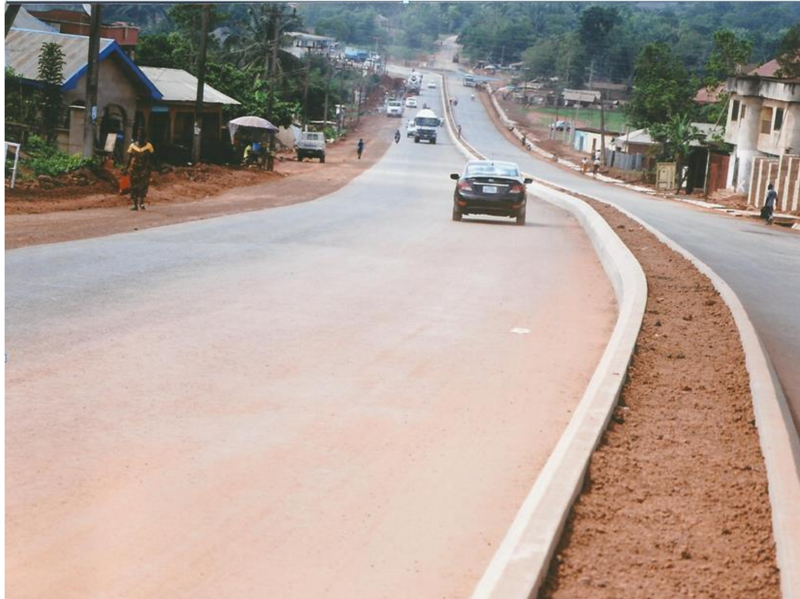
A COMPLETED PORTION OF NSUKKA URBAN ROADS
