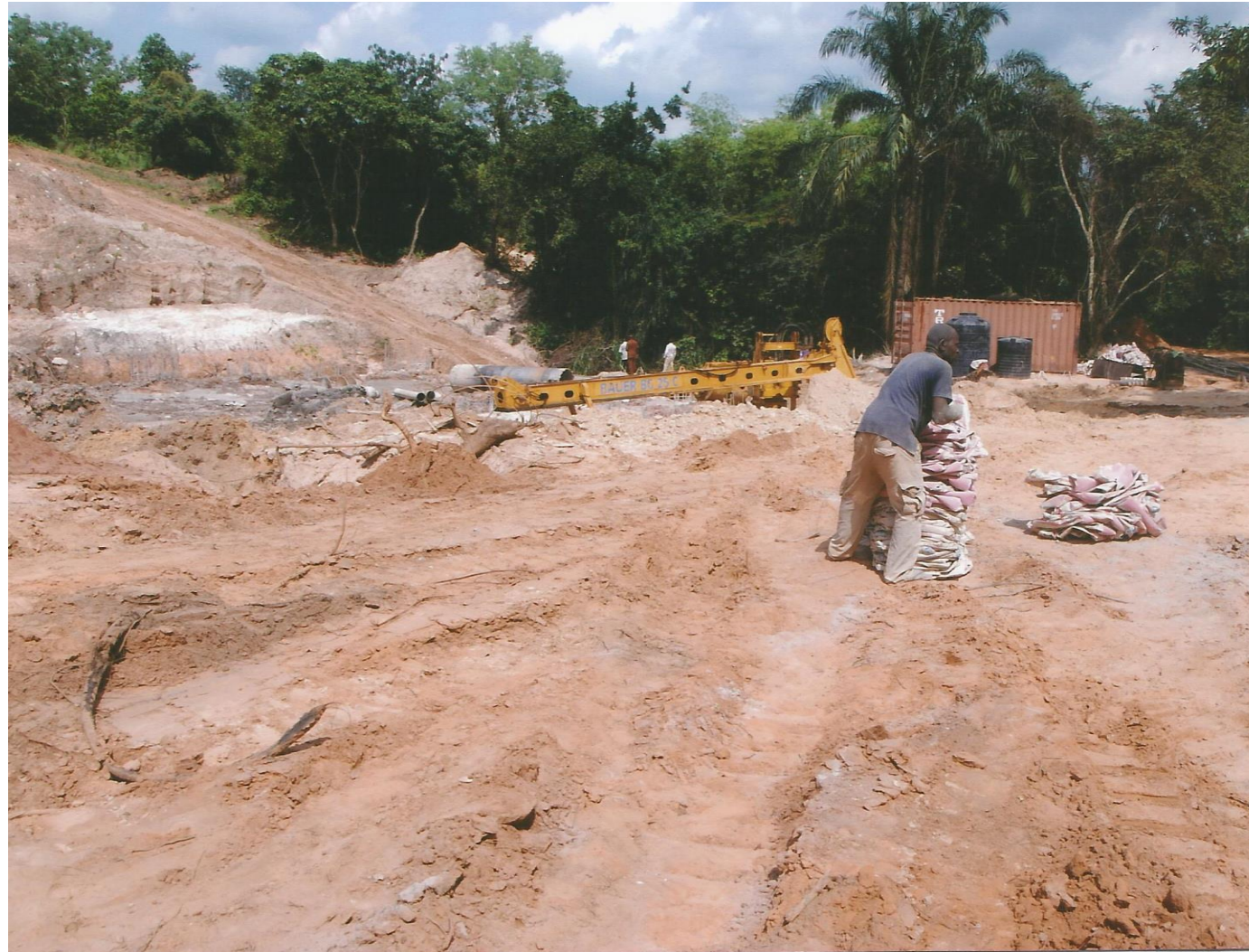
Inyi-Nzu bridge by Ezimo Road under construction
