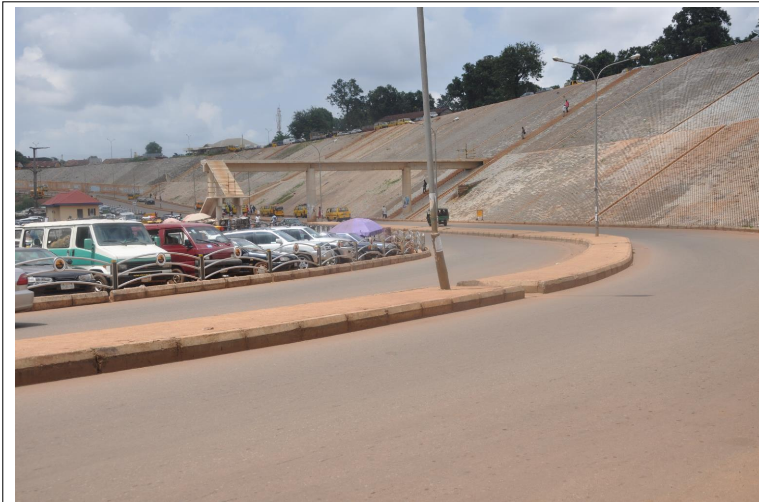
OVERPASS AT AKWATA MAIN MARKET, ENUGU.
