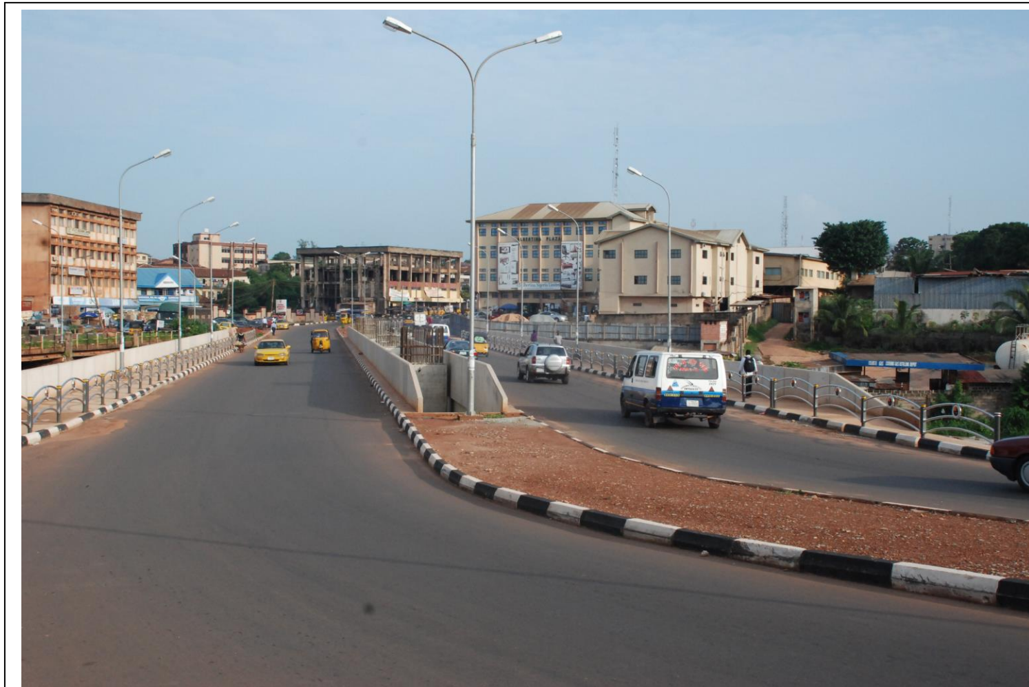
ZIK AVENUE BRIDGE
