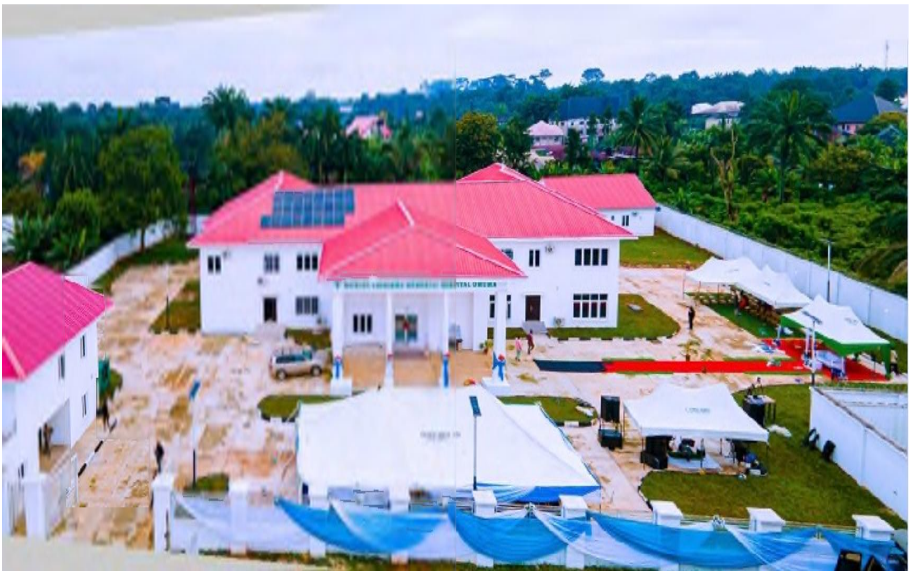
Newly built Ultra Modern General Hospital at Umuokanne in Ohaji Egbema LGA Imo State
