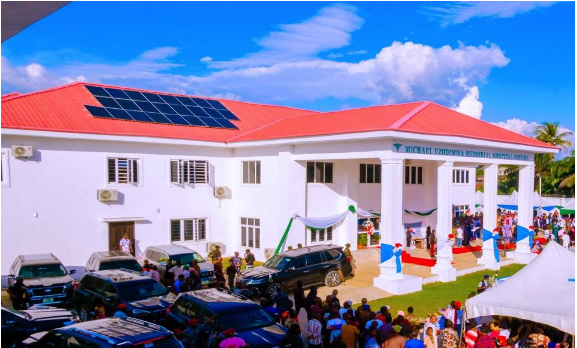
Commissioning of Ultra Modern General Hospital at Omuma Oru East LGA by His Excellency, Dist. Sen. Hope Uzodimma The Executive Governor of Imo State
