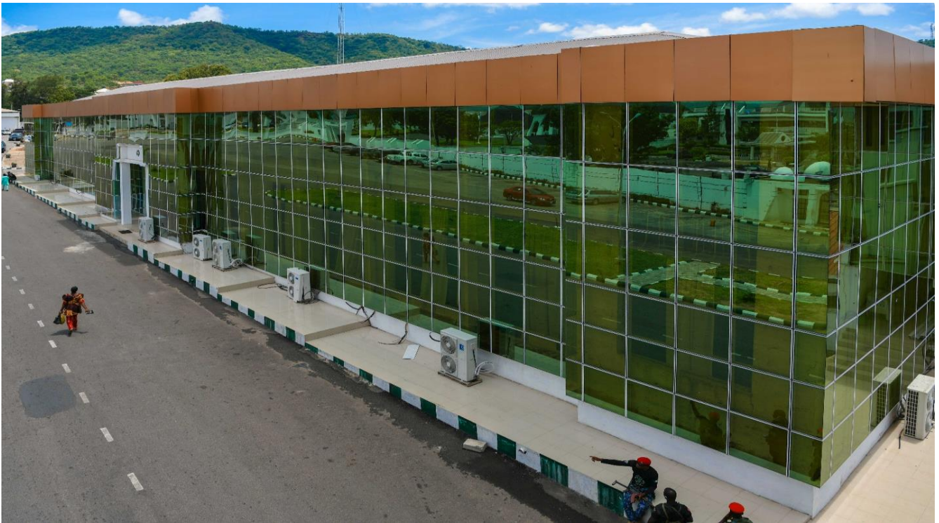
Newly Renovated Glass House, Government House, Lokoja
