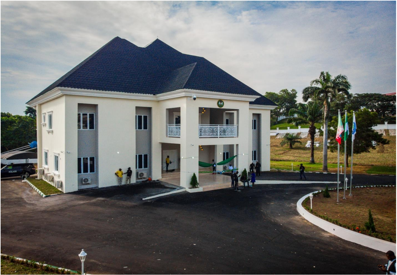
Remodeled Presidential Lodge, Government House, Lokoja
