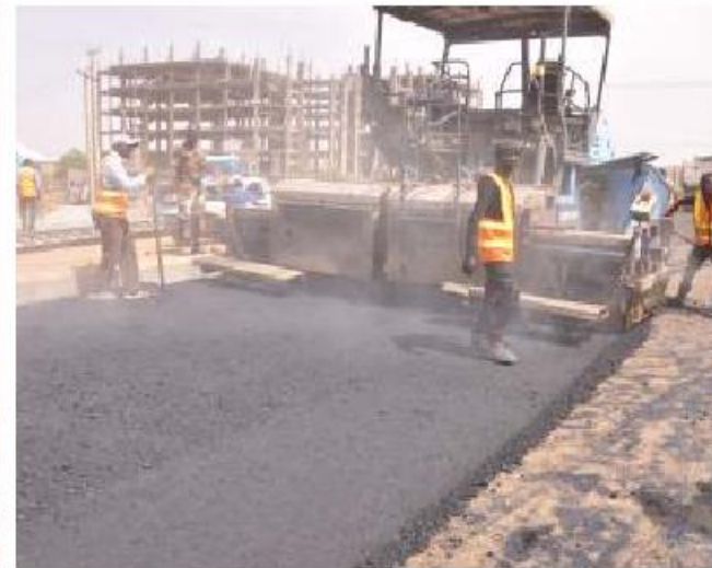
Ongoing Construction of Road Project at Gusau Town
