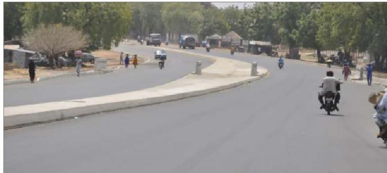
Completed Road Project at Gada Biyu Area in Gusau
