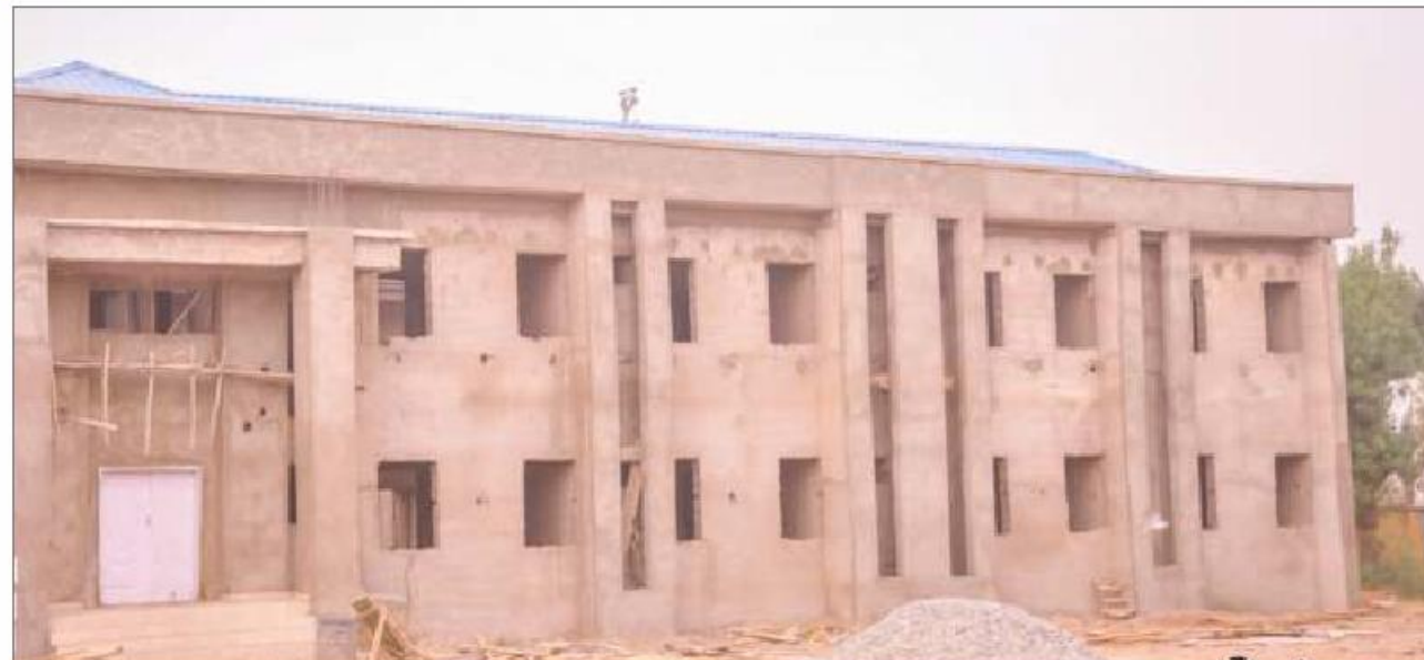
Ongoing Construction Project of Almajiri Schools at Kaura Namoda LGA
