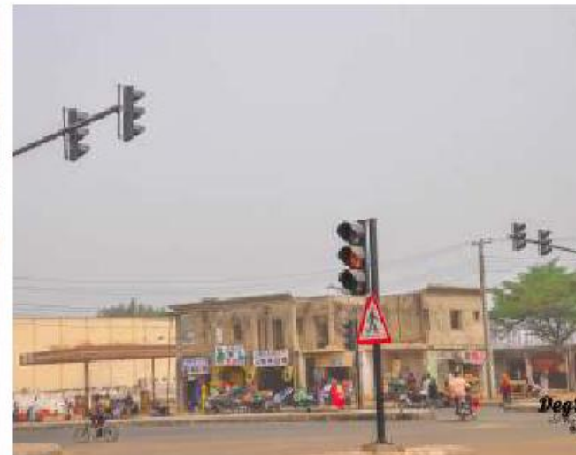
Rehabilitation and installation of Traffic Light at Bello Barau
