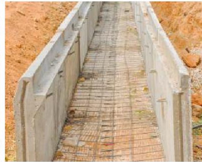
Ongoing Construction of Road Project at Gusau Town
