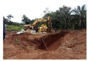
**Picture 9:** Ongoing palliative and culvert works at the Dualization of Akure – Ado Ekiti road project.
