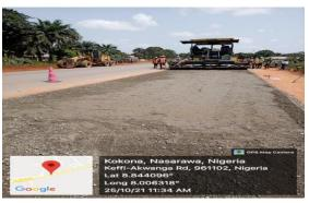
**Picture 10:** Ongoing Bridge Works at Nyanya Axis of Section 1 and laying of stone base at Km15+380 (Sabon Gida Village) – Akwanga Road in Nasarawa State.
